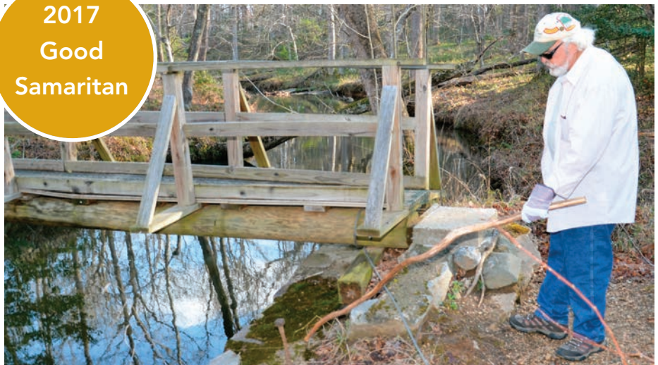
Dorse Counts points to a metal spike, part of the original bridge over Wilderness Run constructed by the Civilian Conservation Corps in the 1930s. The replacement bridge, laid atop utility poles, is anchored by cables to prevent it from washing downstream during a flood.
