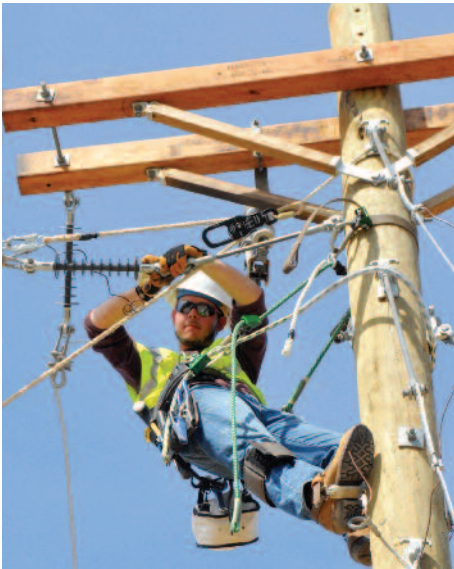
Jackie Lewis Jr. practices pulling conductor in a circuit-construction exercise.
